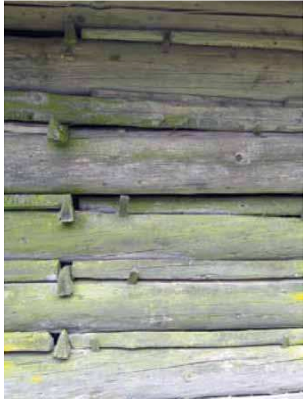
Blockbau Piereni (TN)
