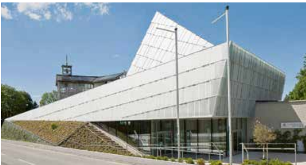
A smart combination of wood and concrete: The Church in Rif is largely energy self-sufficient.
