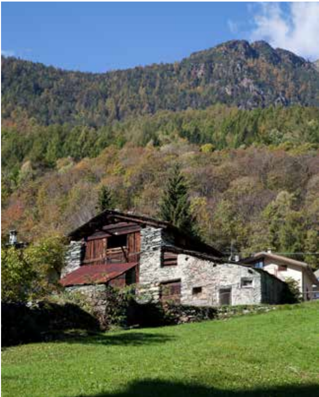
Building in the Municipality of Chiesa in Valmalenco Image: Marco Brigatti
