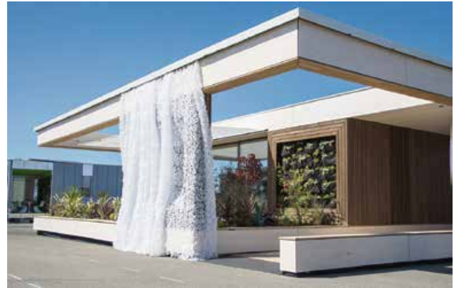
Last year, the LISI House won the Solar Decathlon, a university competition for sustainable construction.
