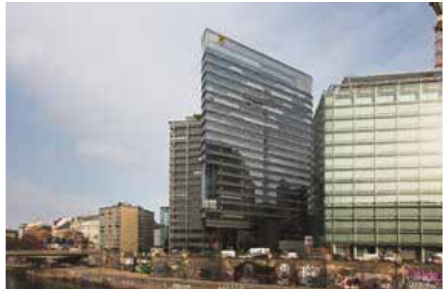
The world's highest passive house additional construction is on the Danube Canal in Vienna.
